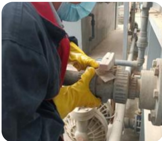
Replacing valve
